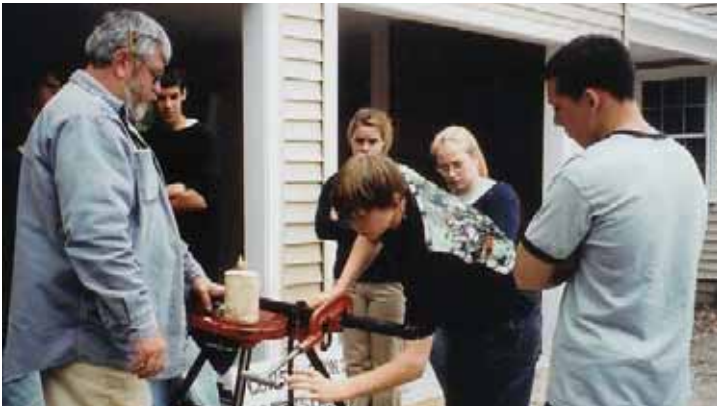
Dave Pelletier and plumbing students at Heather Drive
